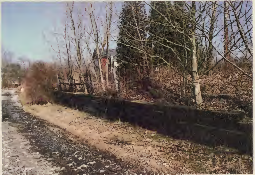
Fig. 122 Railroad ties from the Pickering Valley Line used near the depot in the construction of a retaining wall. The wall is supporting the former embankment that once ran above the gravel road. Photograph by the author, 1995.
